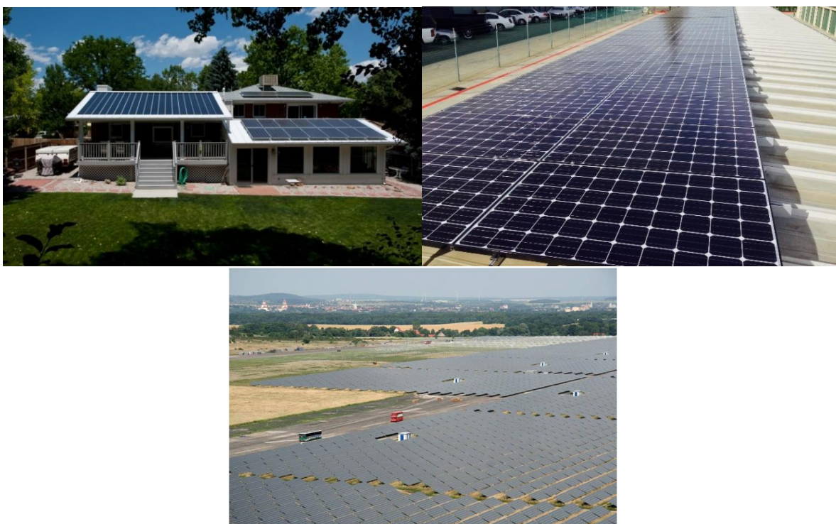
Figure 28. Residential PV (top left), 179 commercial PV (top right), 180 and utility-scale PV (bottom) 181
