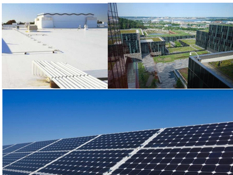
Figure 7. Cool roof (top left); 26 green roof (top right); 27 solar PV (bottom) 28
