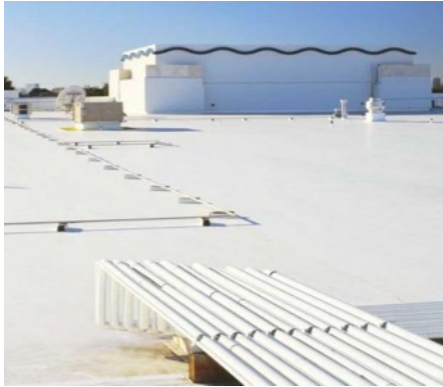
Cool / Reflective Roof
