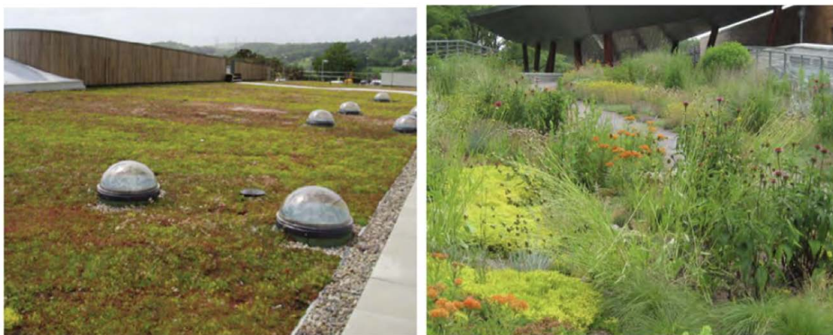
Figure 9.7. Example of extensive green roof (left) and intensive green roof (right) 205
