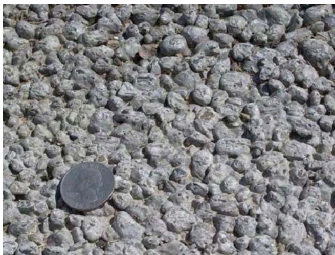
Figure 9.37. Example of pervious concrete pavement surface layer, with quarter to for scale. 405
